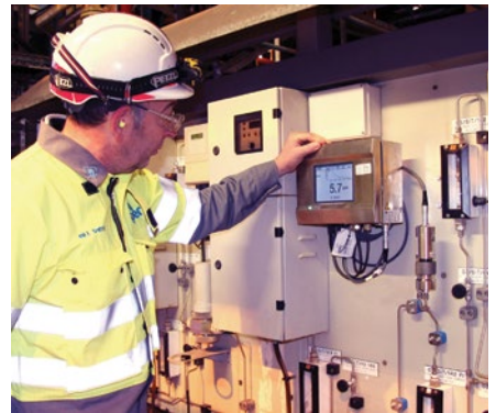
Hach's Orbisphere 410 Controller with a K1100 Optical Dissolved Oxygen Sensor
